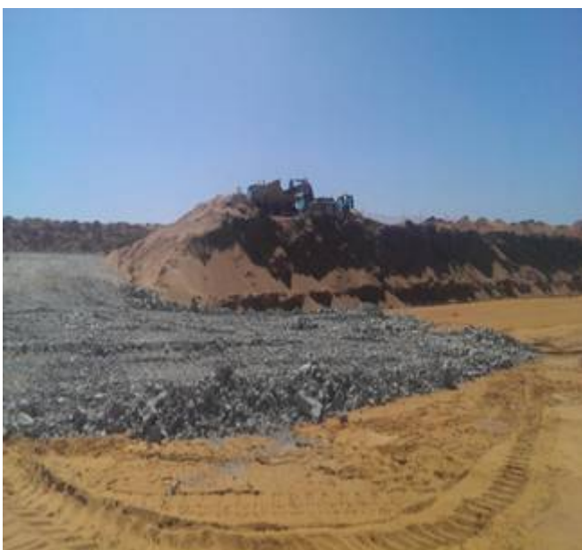
Figure 7.3: Construction of terrace and foundations for substation (Eskom Sere Wind Facility)
