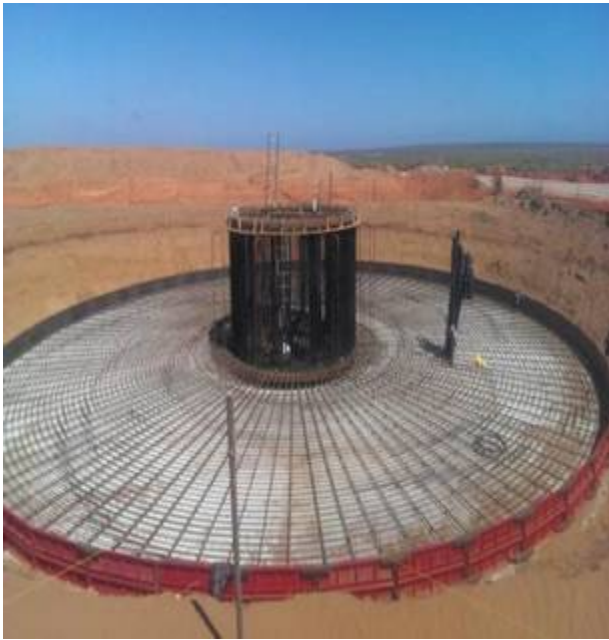
Figure 7.1: Concrete foundation (Eskom Sere Wind Facility)
