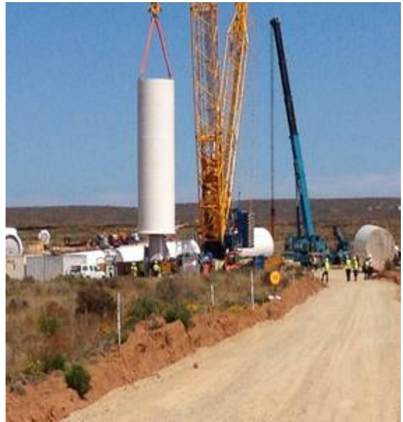
Figure 7.2: Tower sections being lifted (Eskom Sere Wind Facility)
