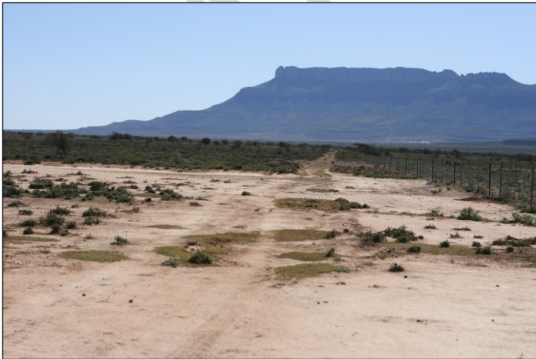
Photo 2-5 Erosion observed on a typical sand road
