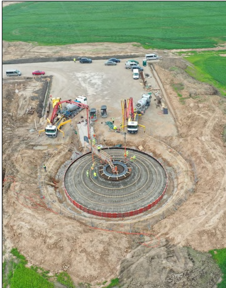
Photo 4-1 Typical Wind Turbine Foundation Construction
