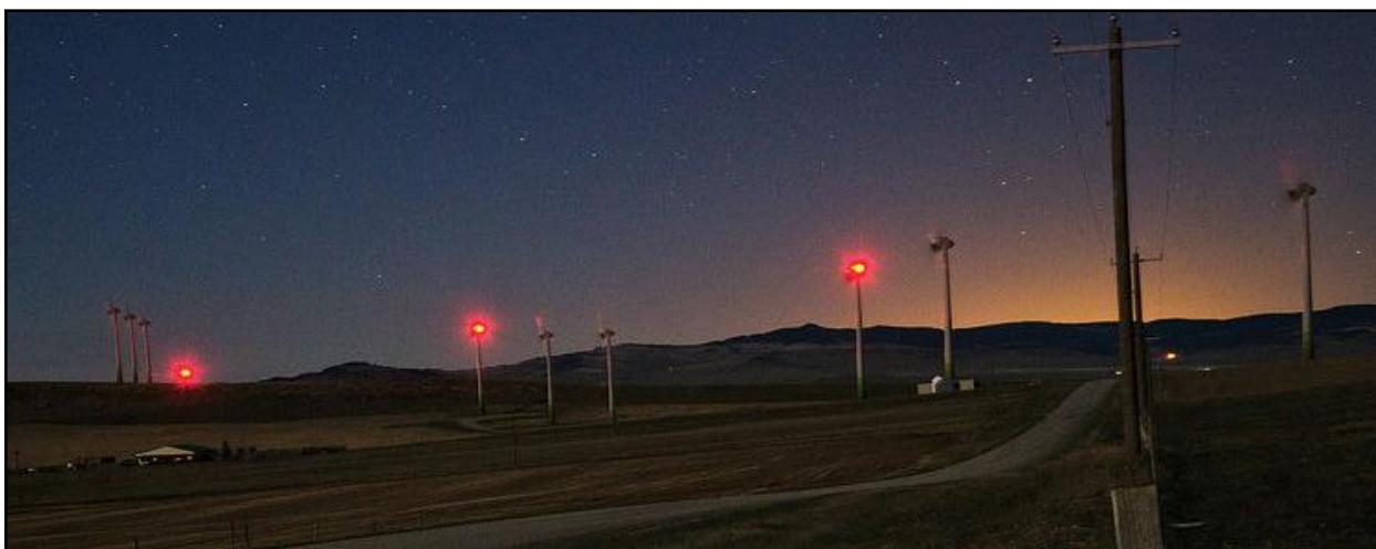
Figure 21: Aircraft warning lights fitted to the wind turbine hubs (Source: http://www.pinchercreekecho.com/2015/04/29/md-of-pincher-creek-takes-on-wind-turbine-lights )
