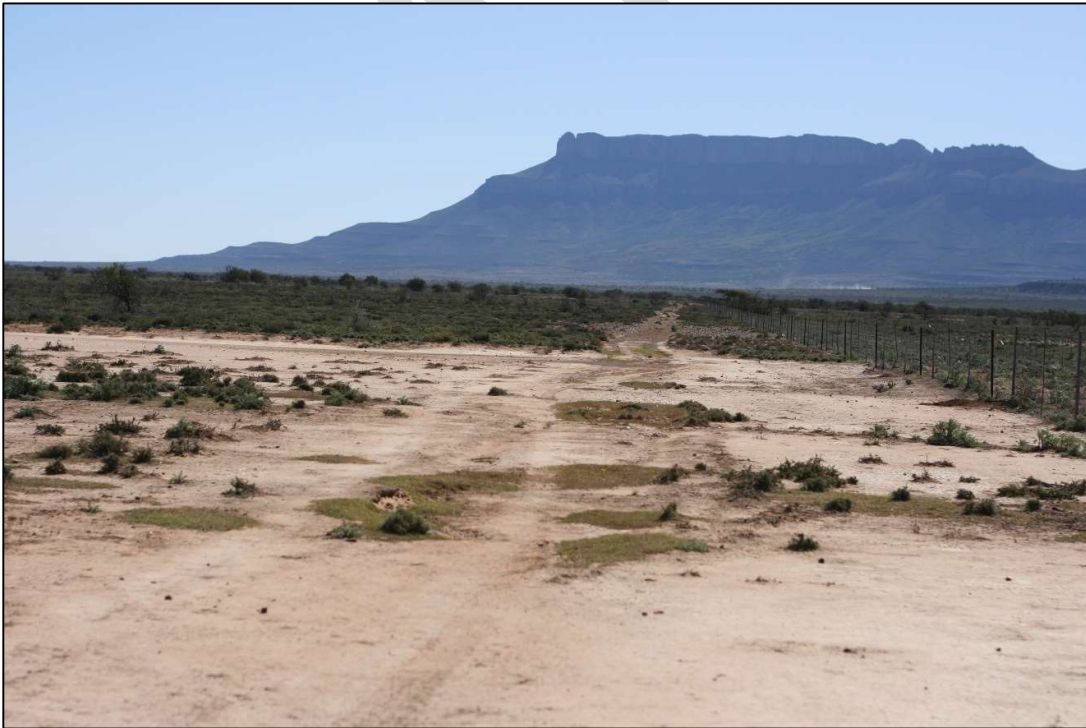
Photo 2-5 Erosion observed on a typical sand road
