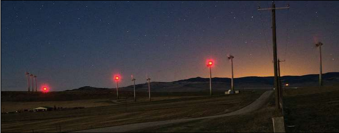
Figure 21: Aircraft warning lights fitted to the wind turbine hubs (Source: http://www.pinchercreekecho.com/2015/04/29/md-of-pincher-creek-takes-on-wind-turbine-lights )
