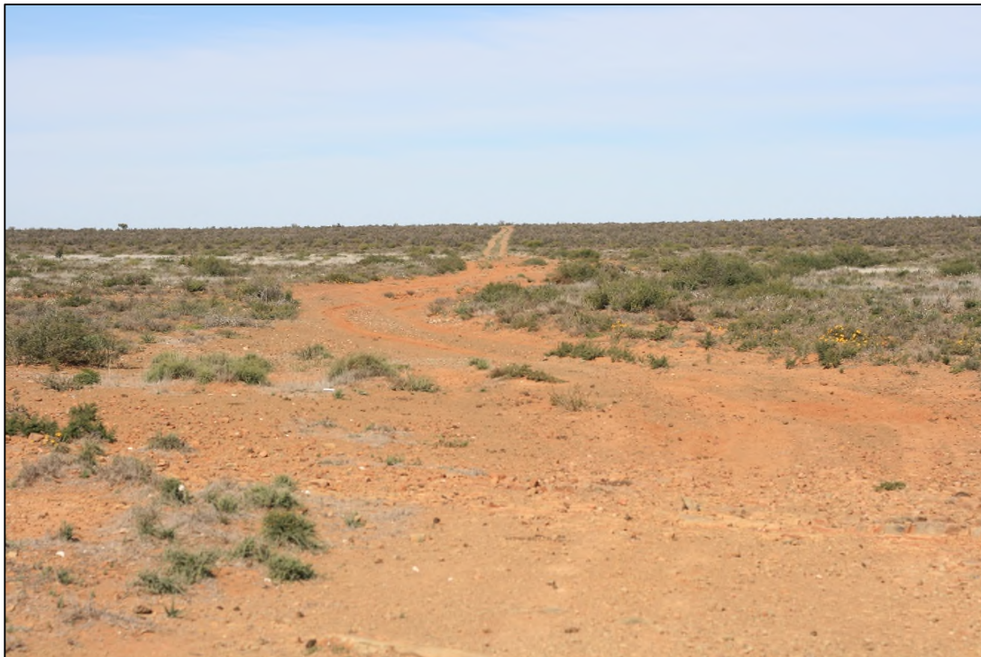
Photo 2-6 Erosion observed on a typical sand road
