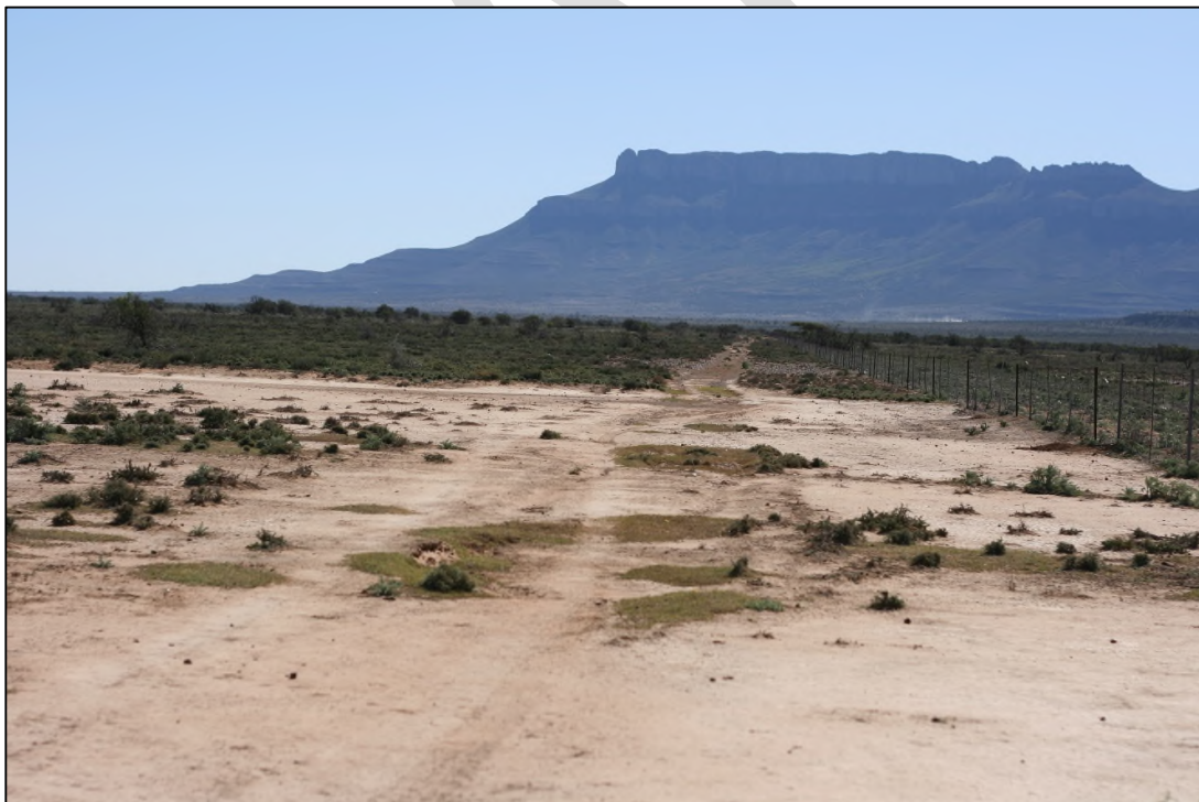
Photo 2-5 Erosion observed on a typical sand road
