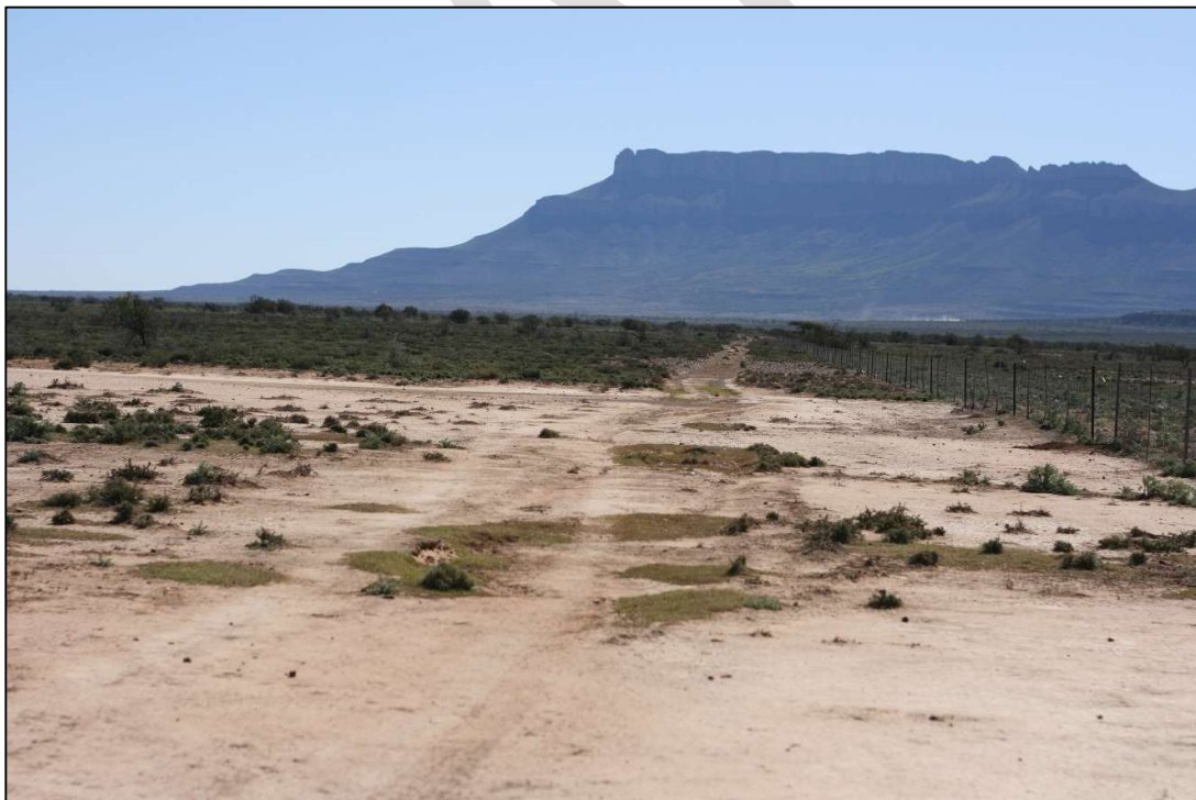
Photo 2-5 Erosion observed on a typical sand road
