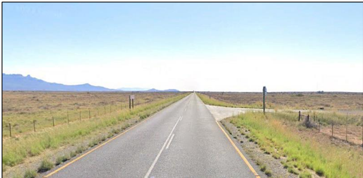
Figure 3-4: R61 at the existing intersection with the internal gravel road (Proposed Site Access)
