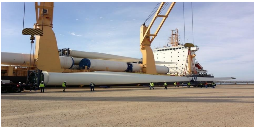
Figure 2-7: Example - Cranes at Port of Entry
