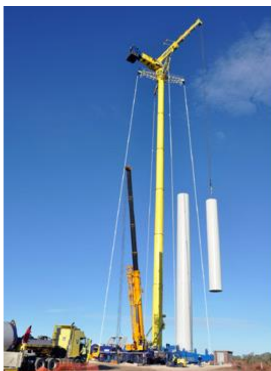
Figure 2-6: Example - Cranes at work
