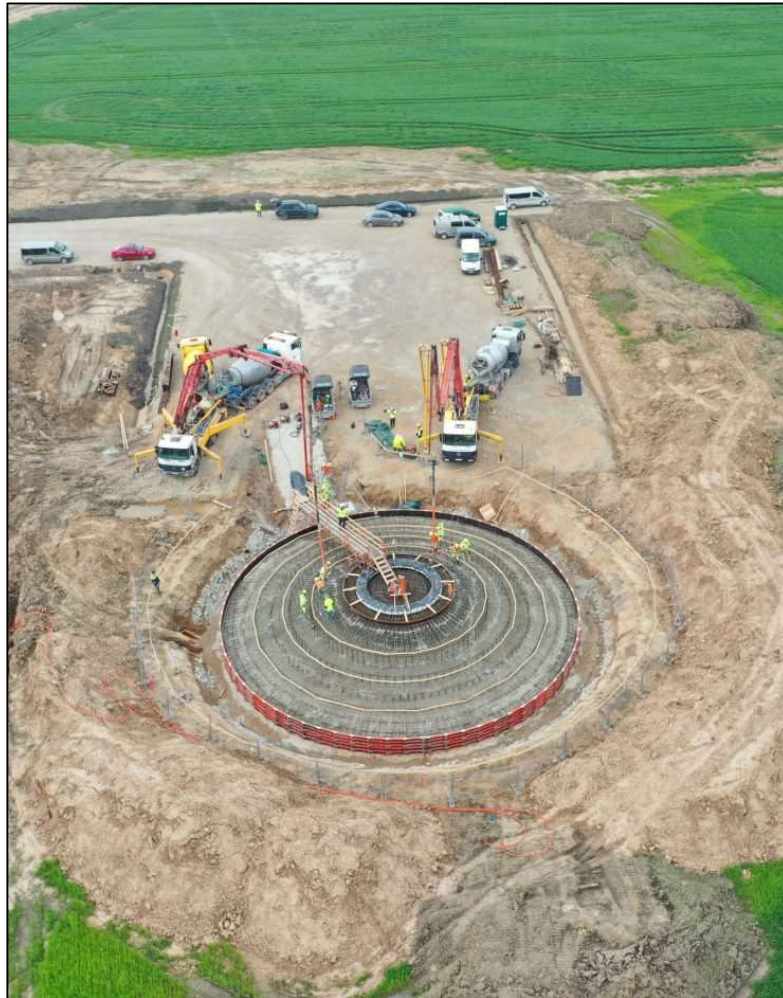
Photo 4-1 Typical Wind Turbine Foundation Construction
