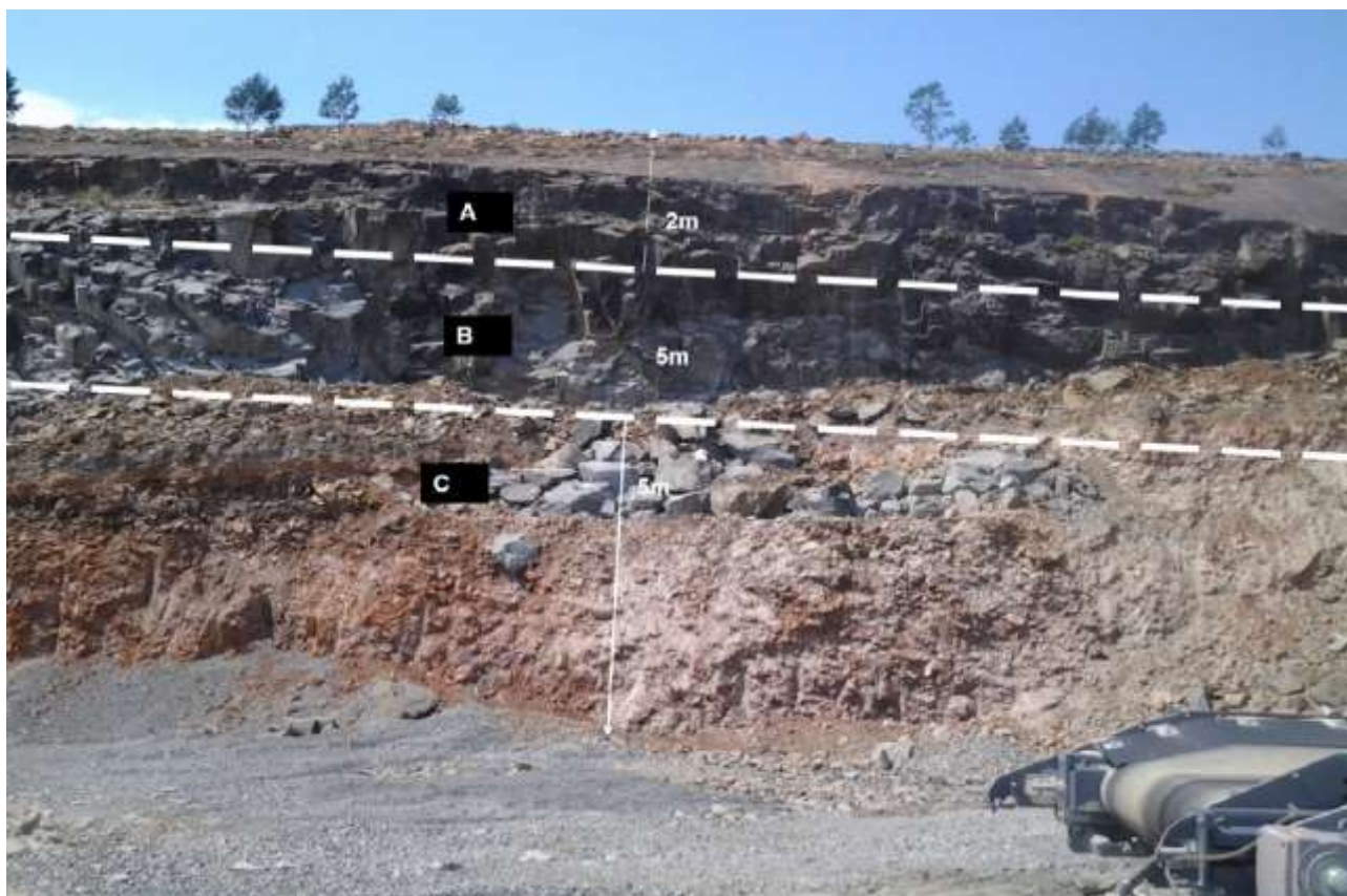
Figure 4: Existing Quarry Mining Cut
