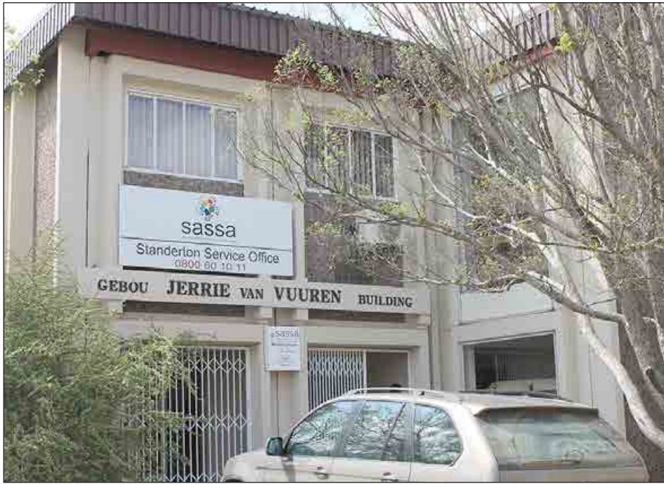
Local SASSA offices at the Gerrie van Vuuren Building on the corner of Paarl and Prinses Street, where beneficiaries can go to update their funeral policies' deductions for 2017.
