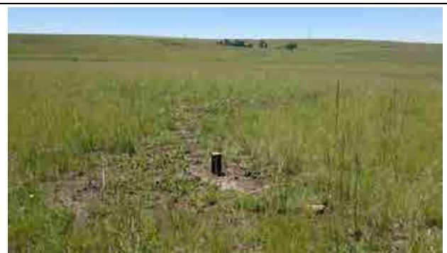
Figure 7: Completed exploration borehole (stand pipe still to be cut below ground level)
