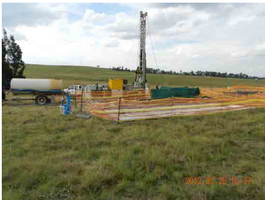
FIGURE 4-9: TYPICAL CORE BOREHOLE DRILLING RIG
