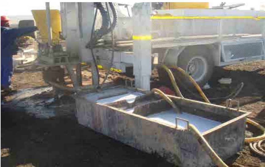
FIGURE 4-13: ABOVEGROUND SKIPS FOR REUSE OF DRILLING FLUID
