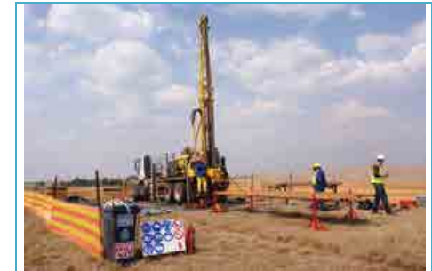
Figure 3: Typical core borehole drilling rig
