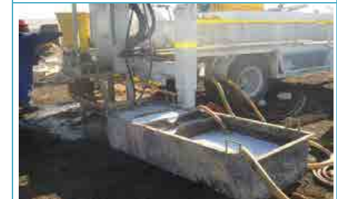
Figure 5: Above-ground skips for reuse of drilling fluid
