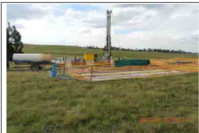
Figure 4: Typical core borehole drilling rig
