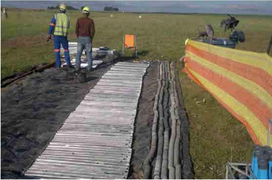
FIGURE 4-10: CORE LAYDOWN AREA
