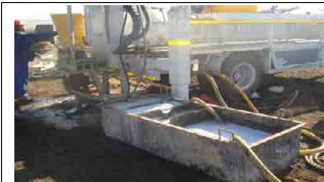
Figure 6: Above-ground skips for reuse of drilling fluid
