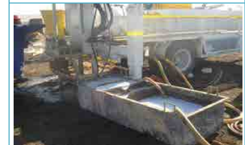
Figure 5: Above-ground skips for reuse of drilling fluid
