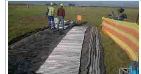
Figure 4: Core laydown area
