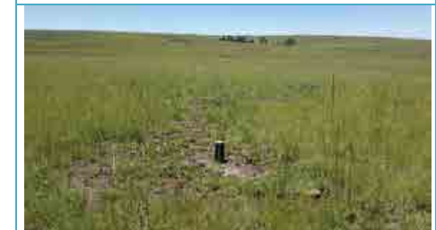
Figure 6: Completed exploration borehole (stand pipe to be cut below ground level)
