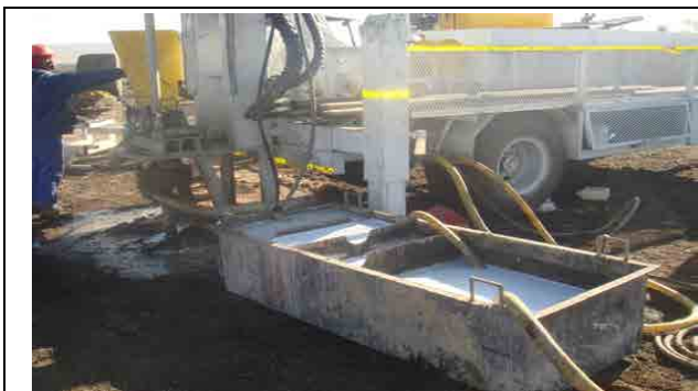
Figure 6: Above-ground skips for reuse of drilling fluid
