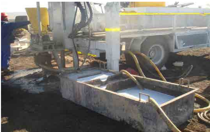
FIGURE 4-13: ABOVEGROUND SKIPS FOR REUSE OF DRILLING FLUID
