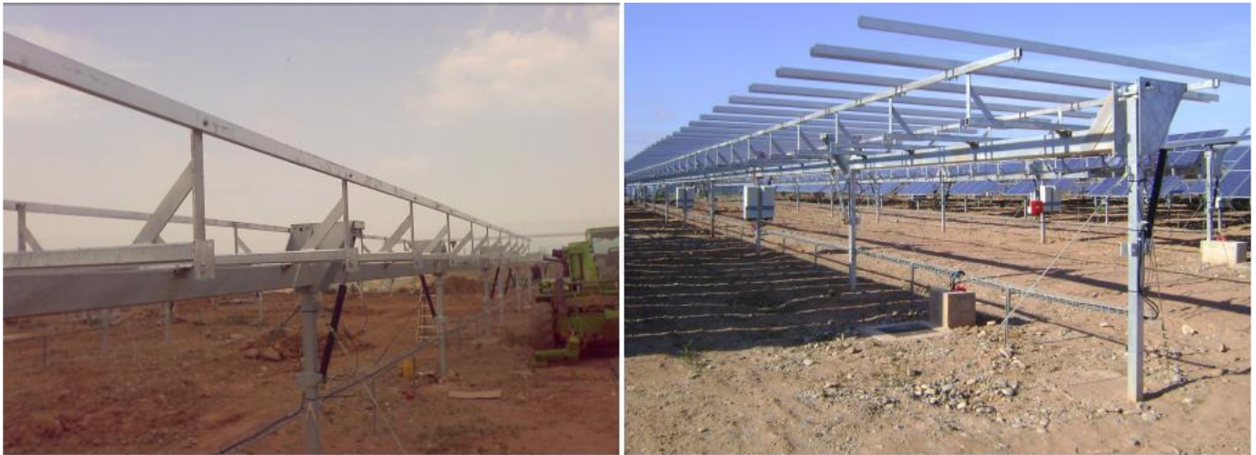
Figure 2.4: Frame, structural details (Photo courtesy of Igeteam, 2011).
