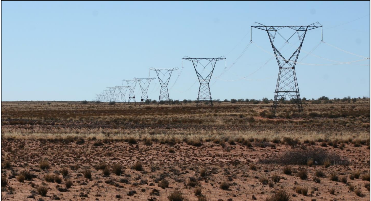
Figure 3. Looking east along the Alternative 1 grid connection corridor from near the N14. The vegetation is Bushmanland Sandy Grassland dominated by Stipagrostis brevifolia . The trees in the distance are Parkinsonia africana .
