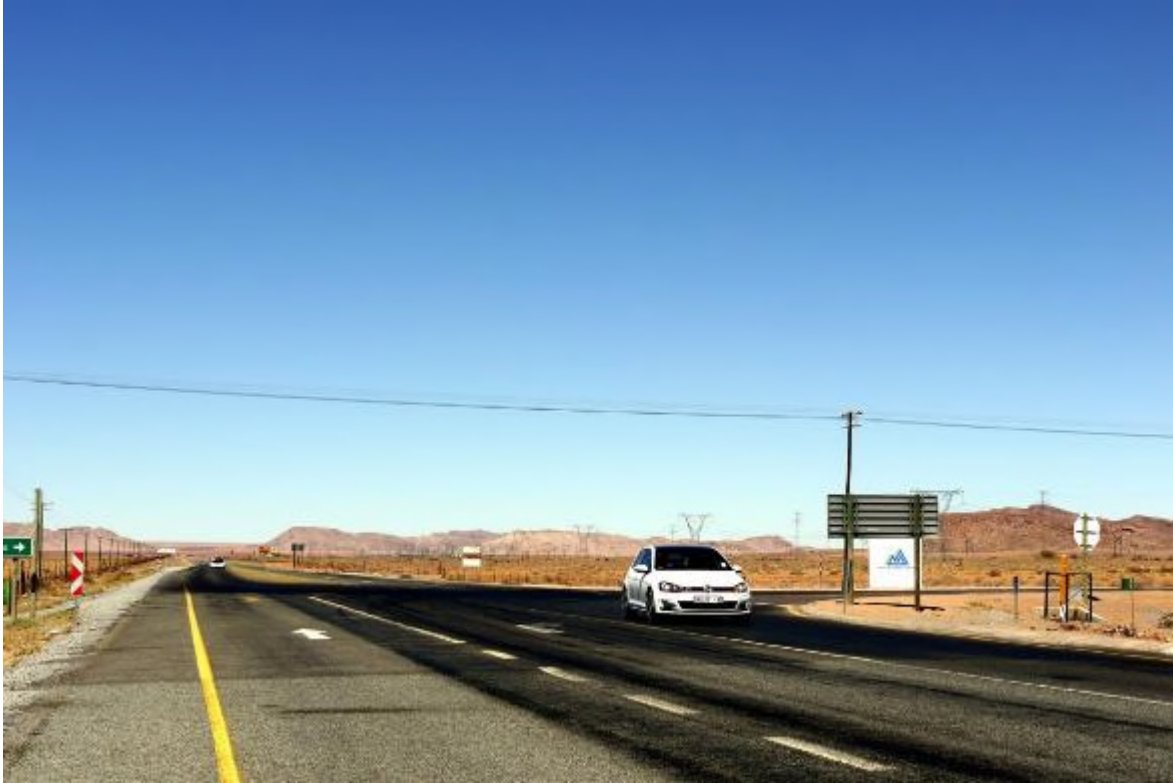
Plate 24, VP 8 – View looking to the south west along the N14 from close to the access road to Aggeneys town. At this position major existing electrical infrastructure is obvious on both sides of the road. Both Power Line Alternative Corridors will be centred on the N14 at this location.
