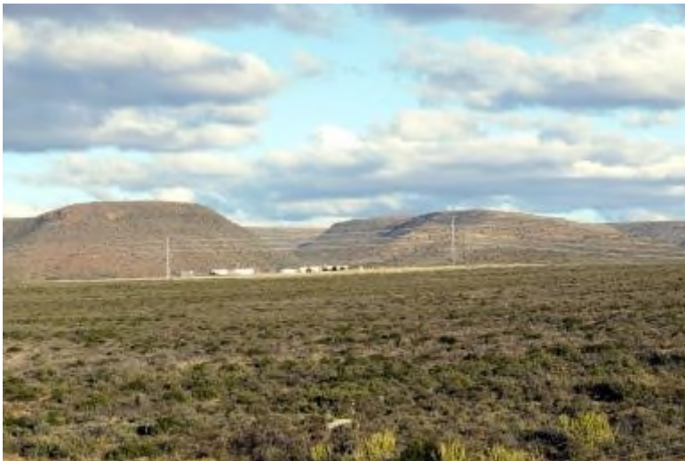
Plate 2, Eskom 220kV Monopole, 40m high.
