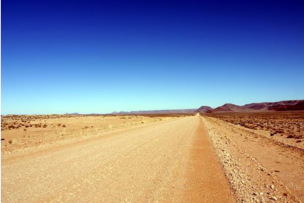
Plate 17, VP1 – View looking to the northwest along the un-surfaced road to the north of the PV project. The viewpoint is immediately adjacent to the proposed Aggeneys 2 PV project which will be located to left of the road. Power line Corridor Alternative 2 will run immediately adjacent to the left side of the road. The area to the north east is currently not impacted by views of power lines.
