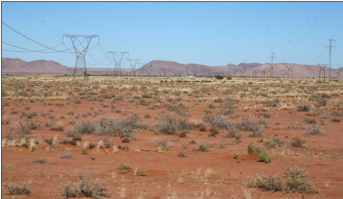
Figure 3. Looking down Corridor Alternative 2 towards the Eskom Aggeneys MTS, showing the typical plains habitat in this section of the route, as well as the large number of power lines already present in the vicinity of the existing substation.
