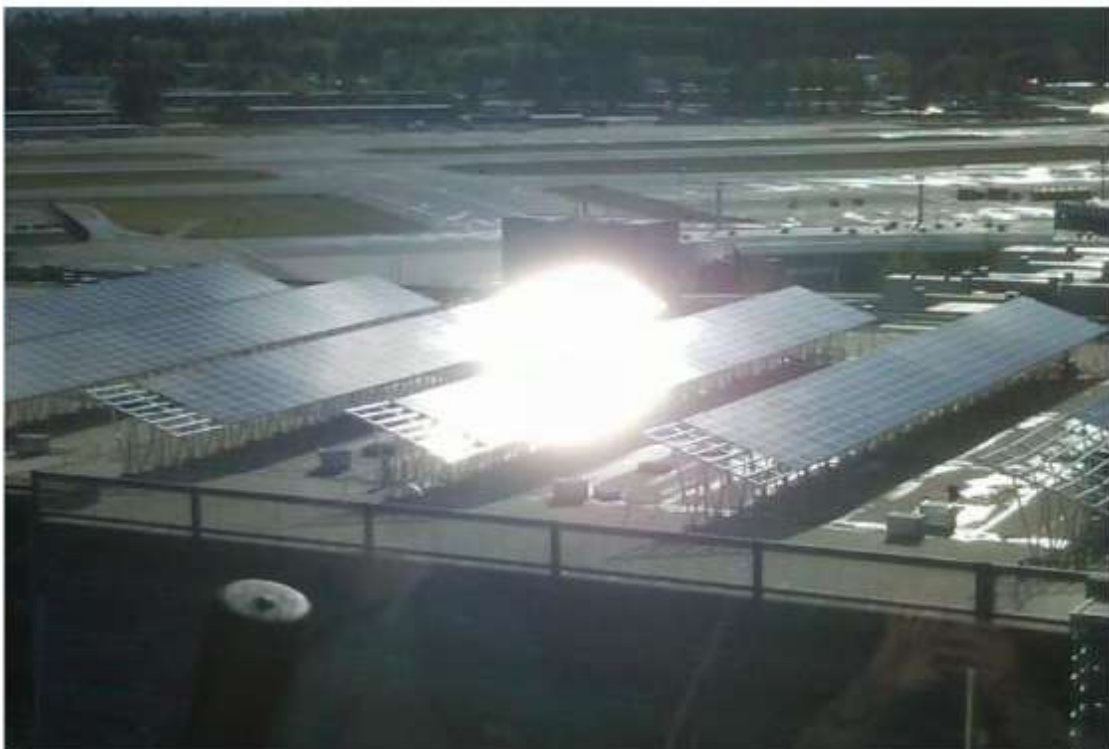
Plate 16 - Glare experienced in the Control Tower at Boston Regional Airport from a PV array
