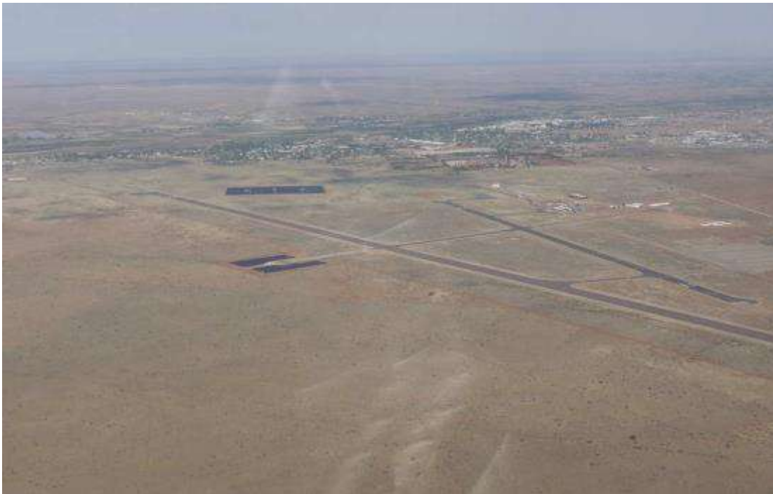
Plate 10 - Existing Solar Arrays at Uppington Airport as seen from the air.
