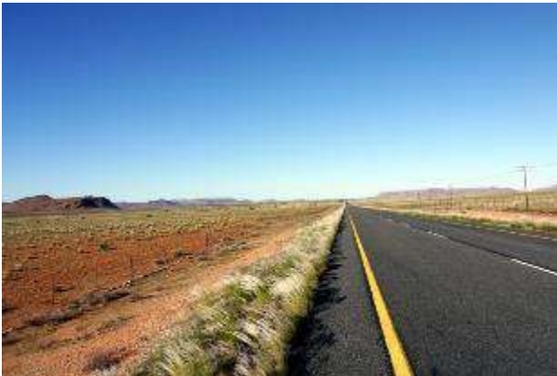
Plate 8, The N14. This is a major regional route that runs to the west of the proposed project area. It is an important regional tourism route
