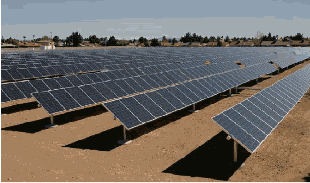
Plate 1. Fixed mounted PV system. Each unit is fixed in place orientated towards the sun's mid-day position. With a single-axis system each row would be placed in a north-south direction and the panels would be moving to follow the sun's position from sunrise to sunset.
