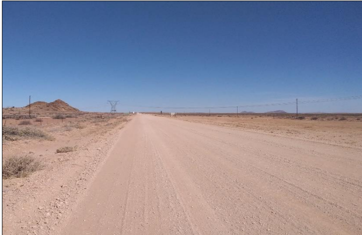
Photograph 4.1: Loop 10 Road during site inspection
