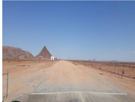
Photograph 5.2: Gravel Access road
