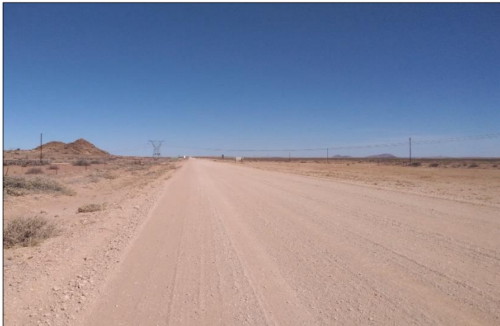
Photograph 4.1: Loop 10 Road during site inspection
