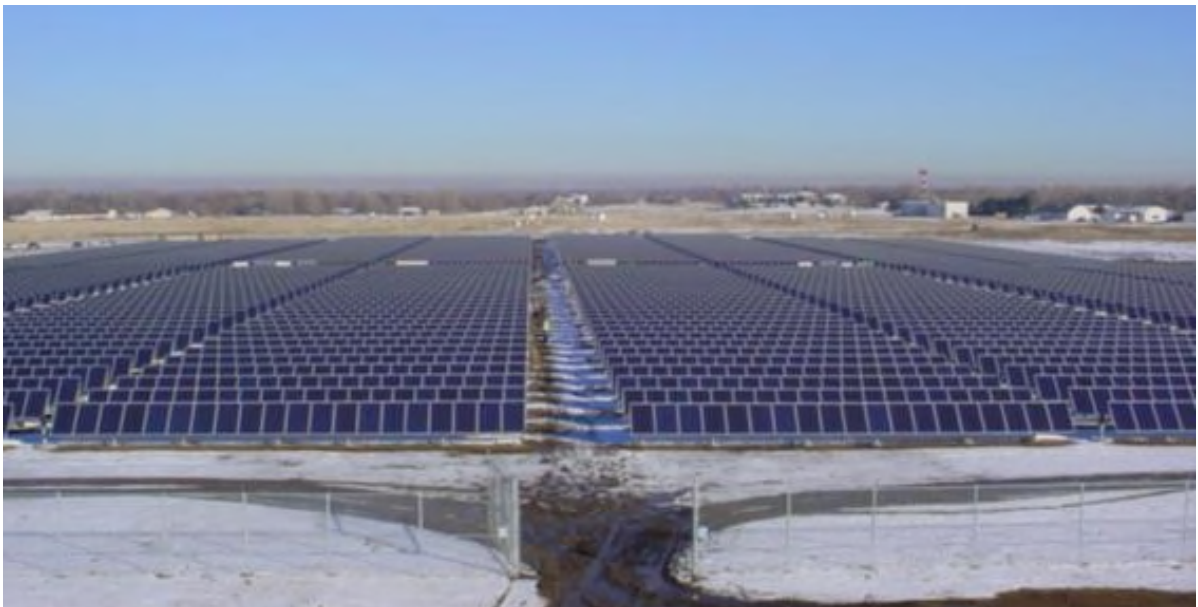
Plate 14 - PV array viewed from above. Note the array rows are read as one and have a similar impact as the roof of a large industrial building.
