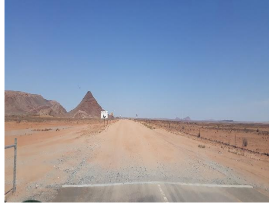
Photograph 5.2: Gravel Access road
