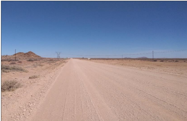
Photograph 4.1: Loop 10 Road during site inspection
