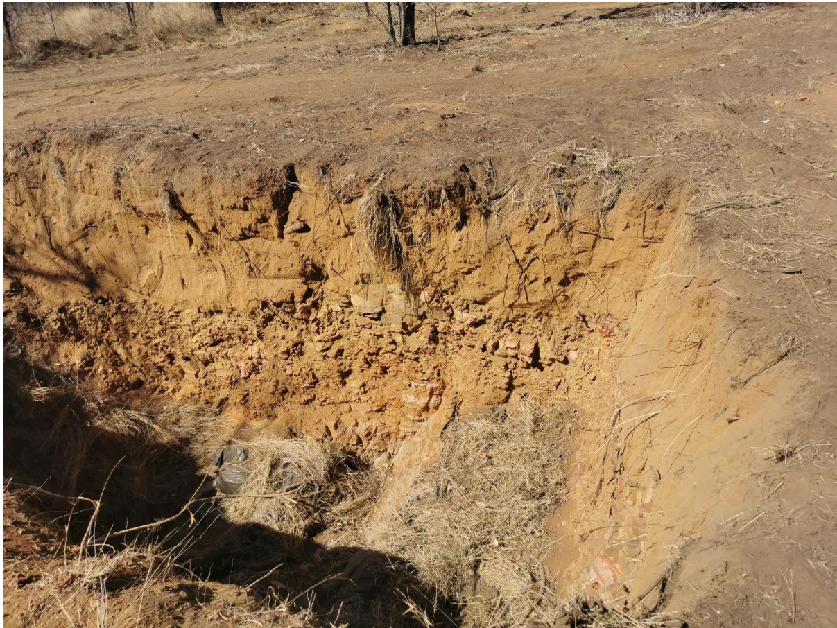
FIGURE 7: EXPOSURE OF SOIL ON WEATHERED SHALE.
