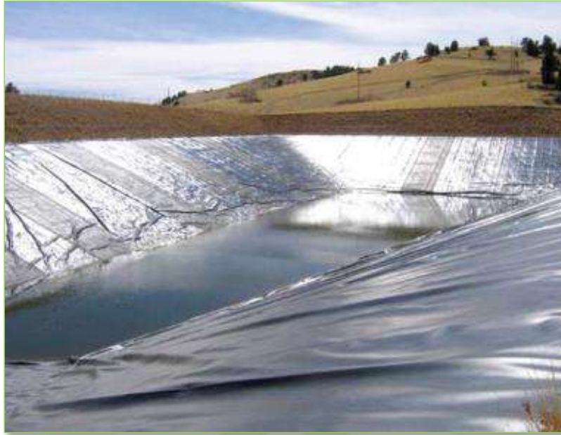
Figure 66: Lined pollution control dam (PCD) illustration
