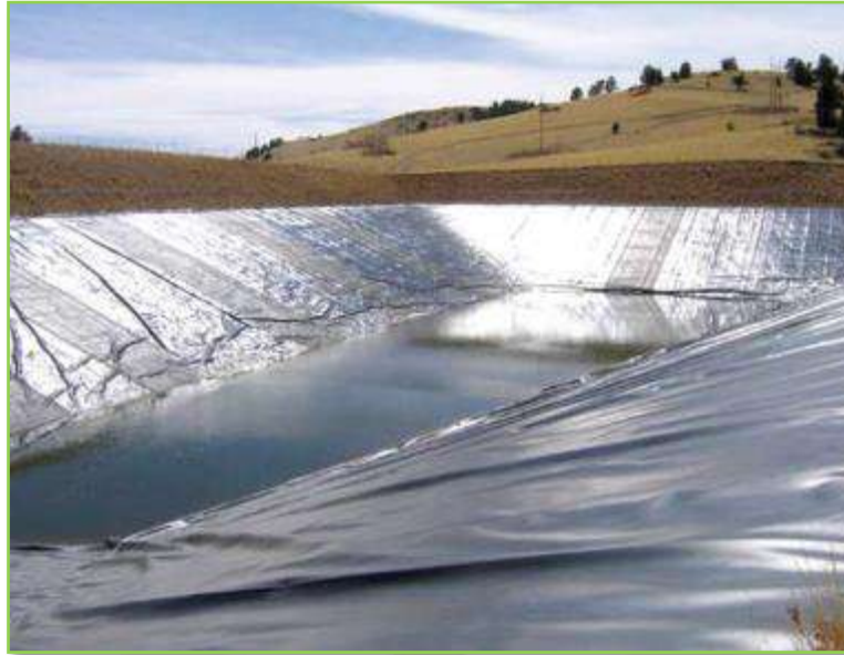
Figure 15: Lined pollution control dam (PCD) illustration
