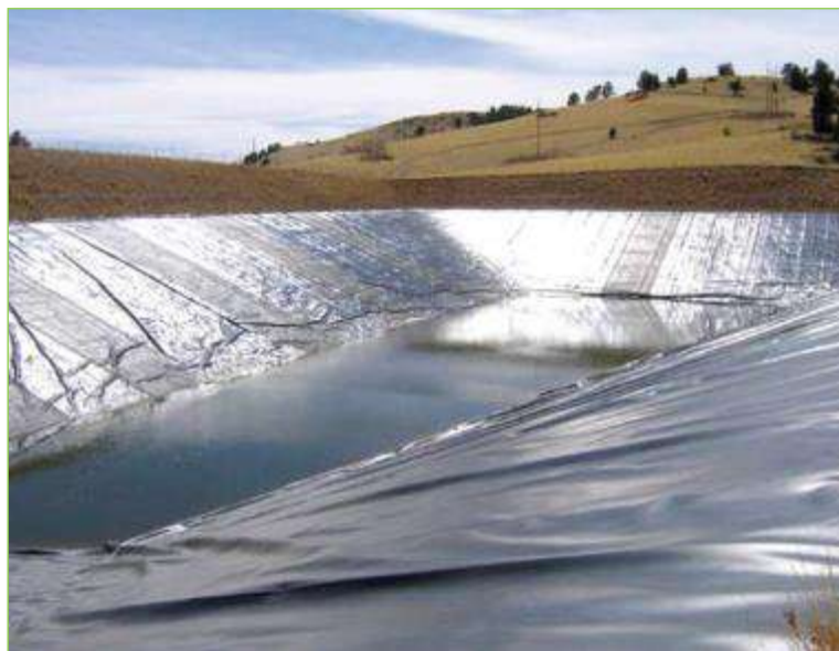
Figure 29: Lined pollution control dam (PCD) illustration
