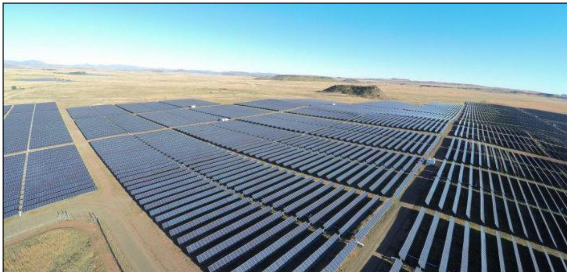
Figure 2: Aerial view of PV arrays. ( Scatec Solar South Africa ).
