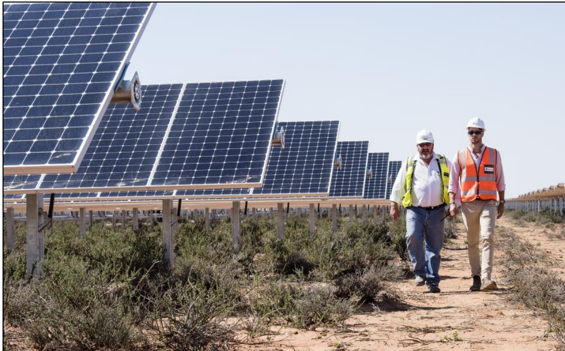
Figure 1: Photovoltaic (PV) solar panels. ( SunPower Solar Power Plant, Prieska ).
