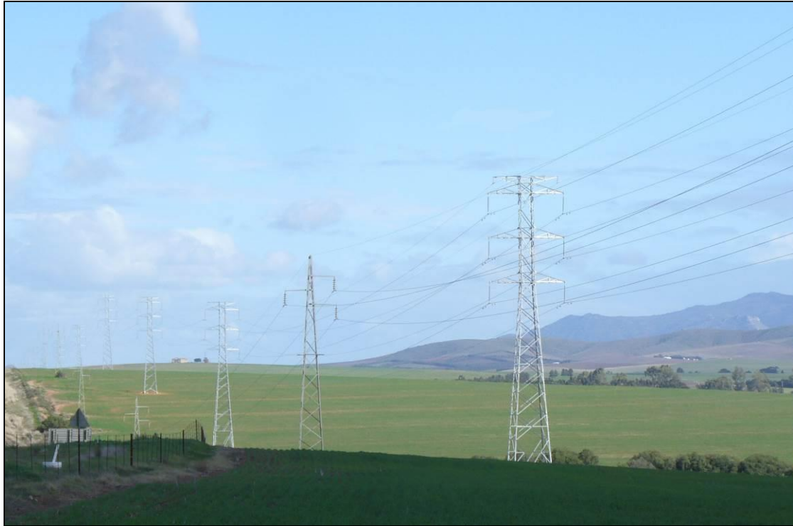
Figure 9: Examples of 132kV overhead power lines.
