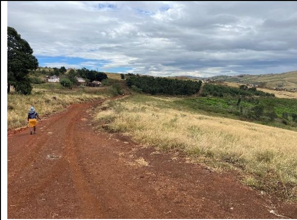
Image 1. The nature of the existing track proposed for upgrade near the start point.
