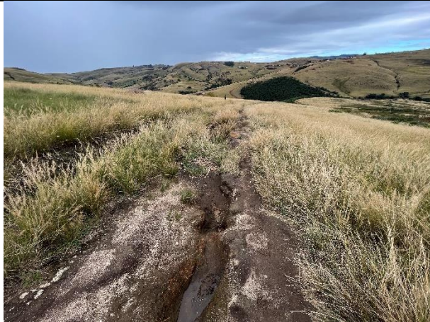
Figure 18. Image looking south west showing the existing track and erosion gulleys on the northern approach to the Madiyana River valley.
