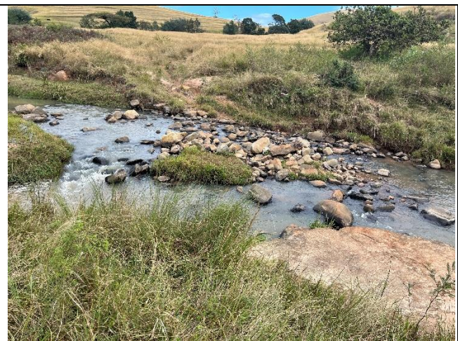
Plate 2. Image looking north overlooking the Proposed road bridge and road alignment at the Madiyana River watercourse crossing towards the mid-point of the road construction.
