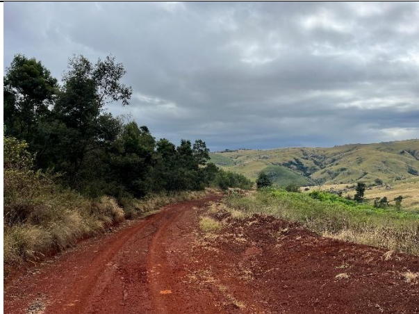
Figure 12. Image looking north showing the existing track proposed for upgrade. Note track surface in poor condition and slippery when wet.
