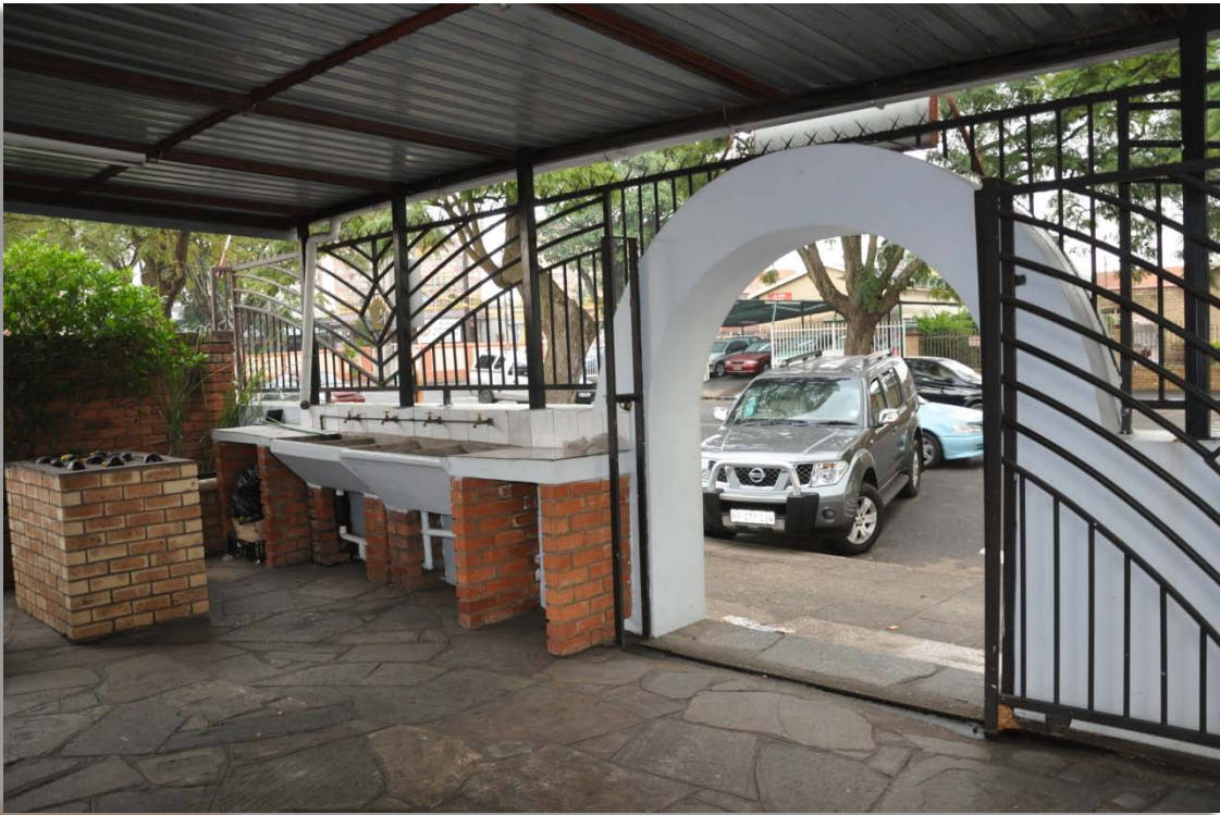
Existing Boundary wall/ Entrance
