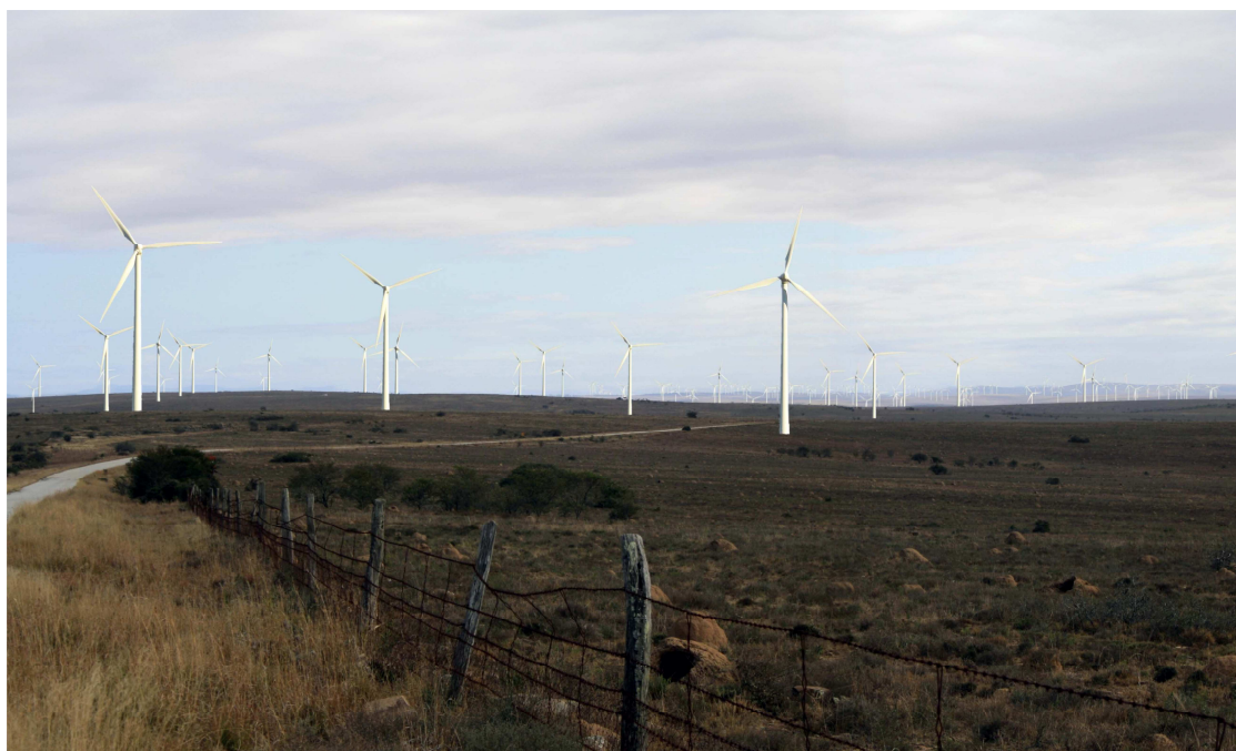
Figure 6.8: View from the R350 as it enters the site from the south. This position is very close to the closest turbines and is indicative of what will be seen from the western sections within the facility footprint. This view includes the cumulative view combining both proposed Amakhala Emoyeni Wind Energy Facility and approved Cookhouse Wind Energy Facility turbine positions.
