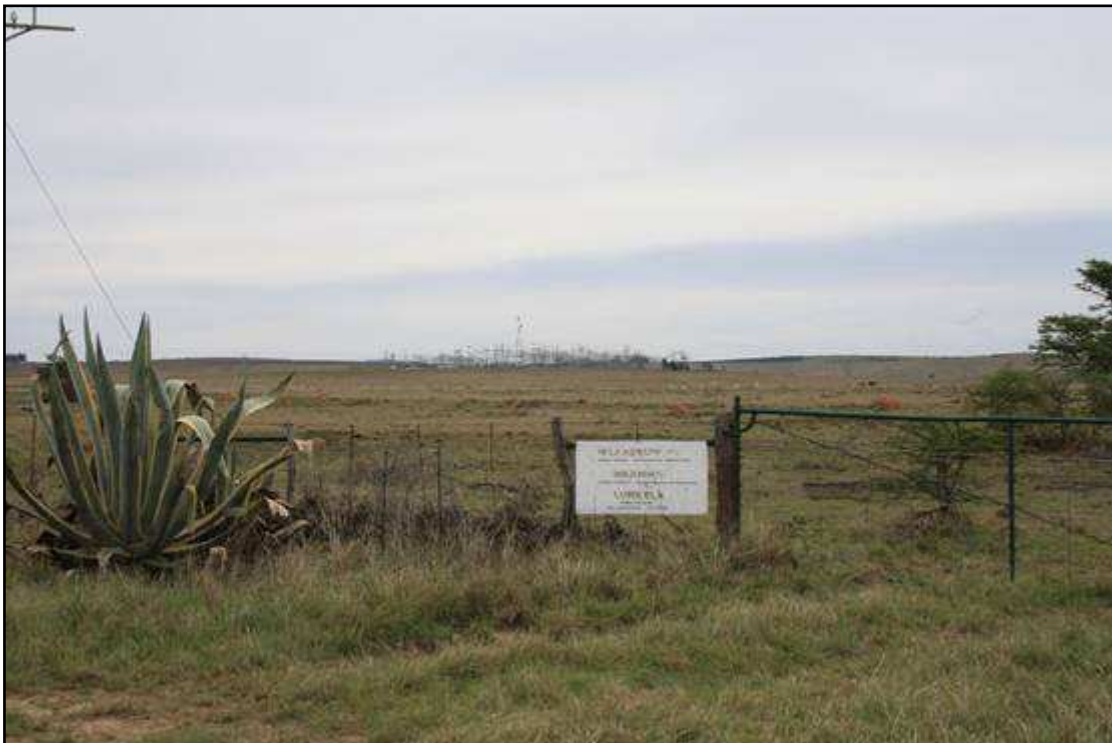
Figure 3: General environment surrounding the Poseidon substation (taken from within the proposed development area).
