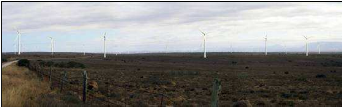
Figure 8a: Panoramic overview from Viewpoint 1 also including ROD approved Cookhouse turbines.
