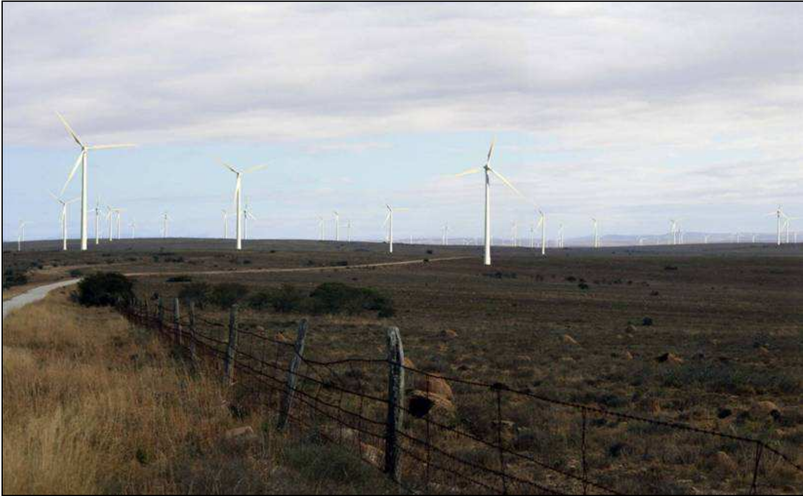
Figure 7c: View 1a (enlarged photograph section from Viewpoint 1).
