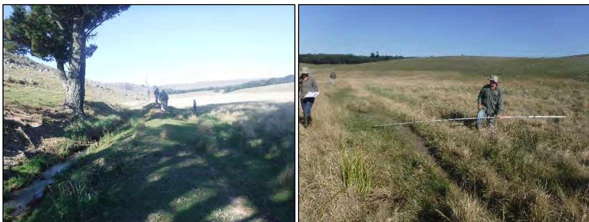
Figure 4.6 The straightened channel running down the left-hand bank of the wetland (left), and a berm limiting diffuse flows through the wetland (right)
