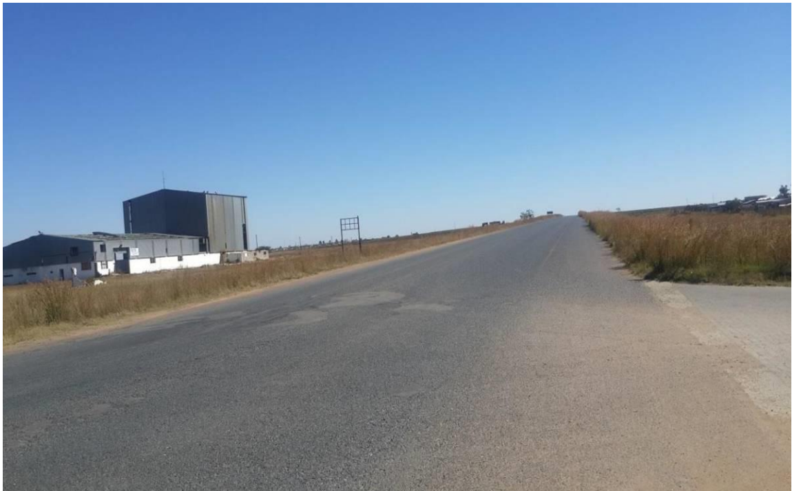
Old milling structure on site
