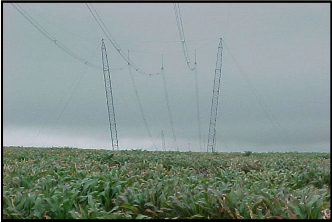
Figure 10: Cross Rope Structure
