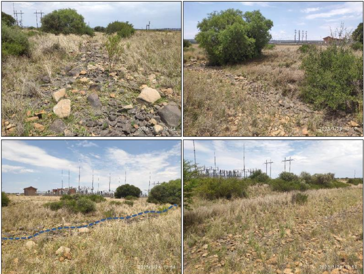
Figure 37: Rocky streambank of the non-perennial steam (top) and a view of the substation from west of the non-perennial stream (bottom) (Vegetation Review, 2023)
