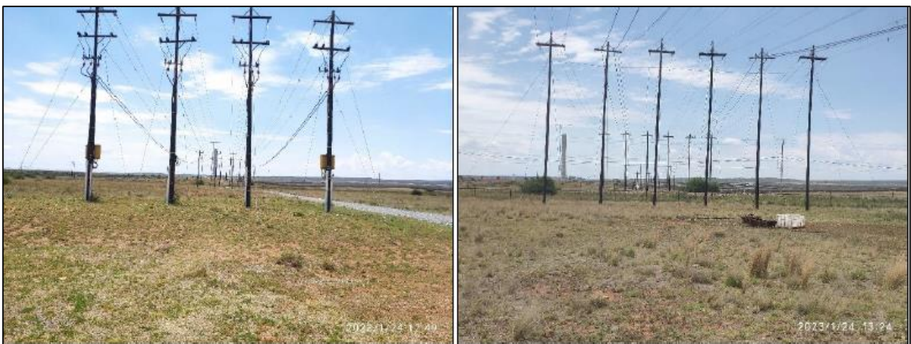
Figure 39: Vegetation under the southern extent of the powerlines (Vegetation Review, 2023)
