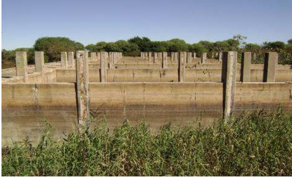
View of the abandoned waste water treatment works concrete structure noted on the proposed site.
