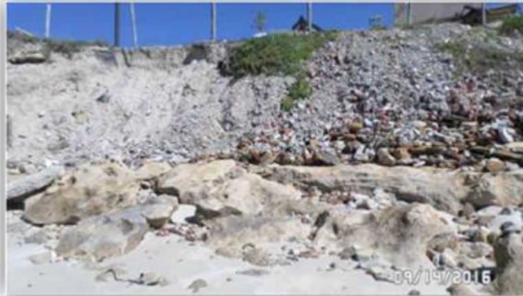
Figure 5: Arniston harbour embankment.
