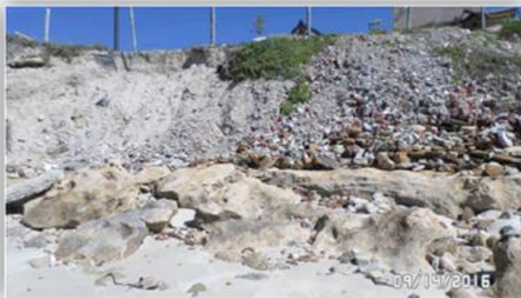
Figure 5: Arniston harbour embankment.
