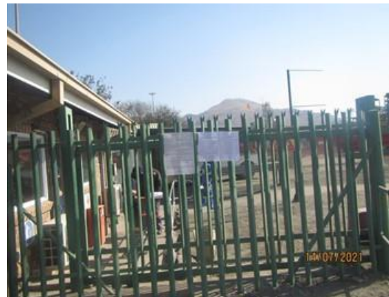
Plant Entrance (Project 4 and 5)
