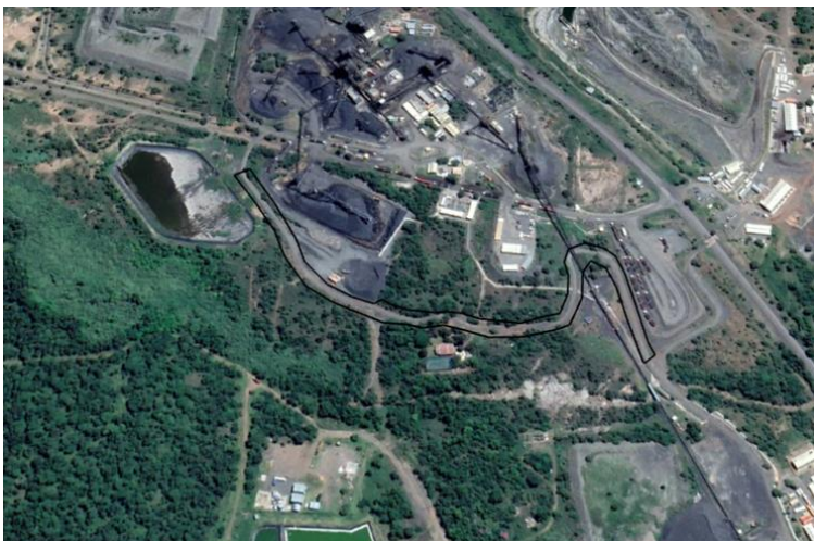
Figure 4: Widening of access road
