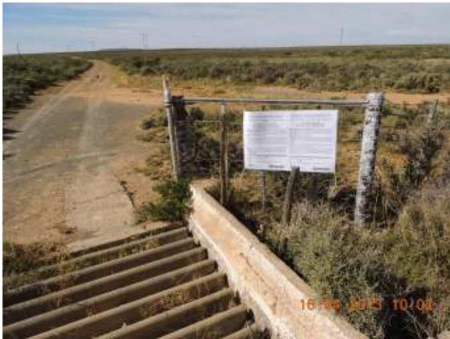
Site notice placed on the gate (30°35'56.32"S; 24° 2'32.58"E)
