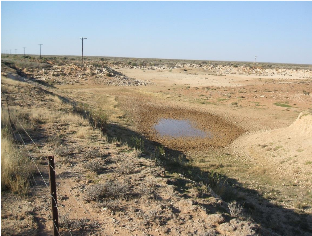
Figure 9: Large Borrow Pit on R357 approximately 2.6km from the Kronos sub-station
