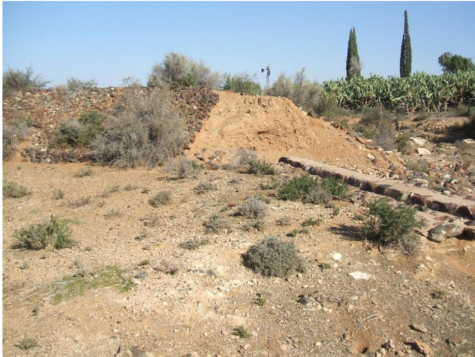
Figure 12: Hoekplaas farm dam wall
