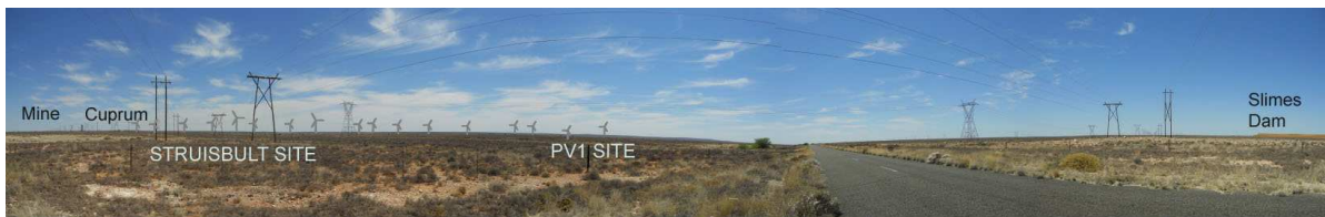
Fig 5.11 View of the proposed Preferred and Alternative layouts for Struisbult, from the road to the Mine, showing the relationship with the proposed PV1 installation and the proposed WEF, (Plan 8).
