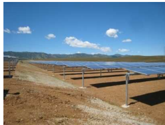
Fig 2.3. Image of Ray tracker utility scale solar tracker installation. Tech Option 1 Source Mulilo
