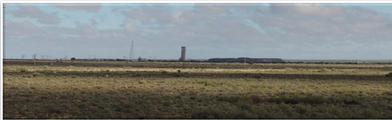
Figure 11: View of existing mining infrastructure of Copperton Mine
