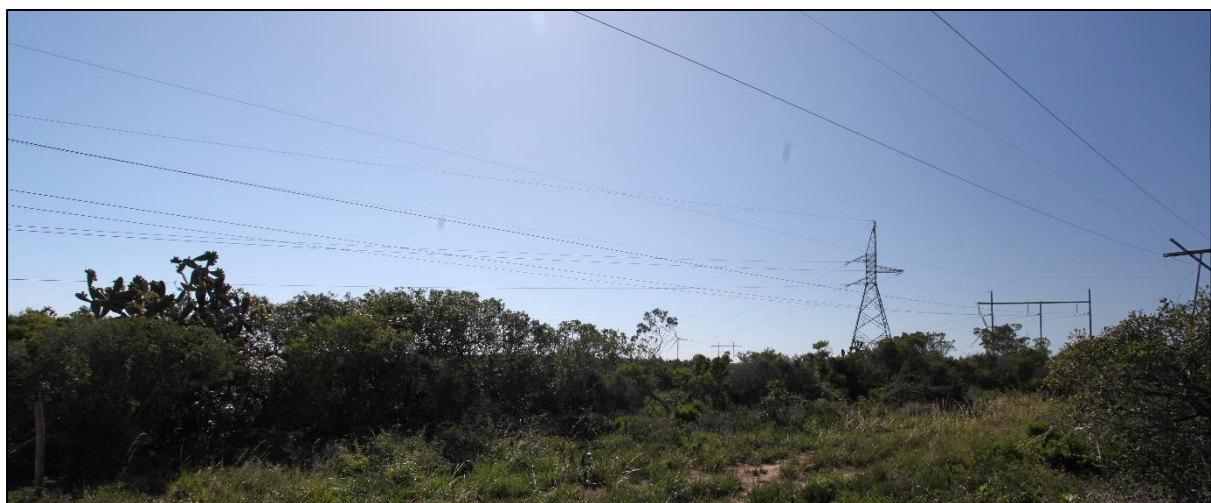
Figure 16: View from a gravel road traversing the southern portion of the proposed OHPL. The existing overhead powerline is clearly visible from this vantage point, as such the proposed OHPL will have a higher visual impact at this point.
