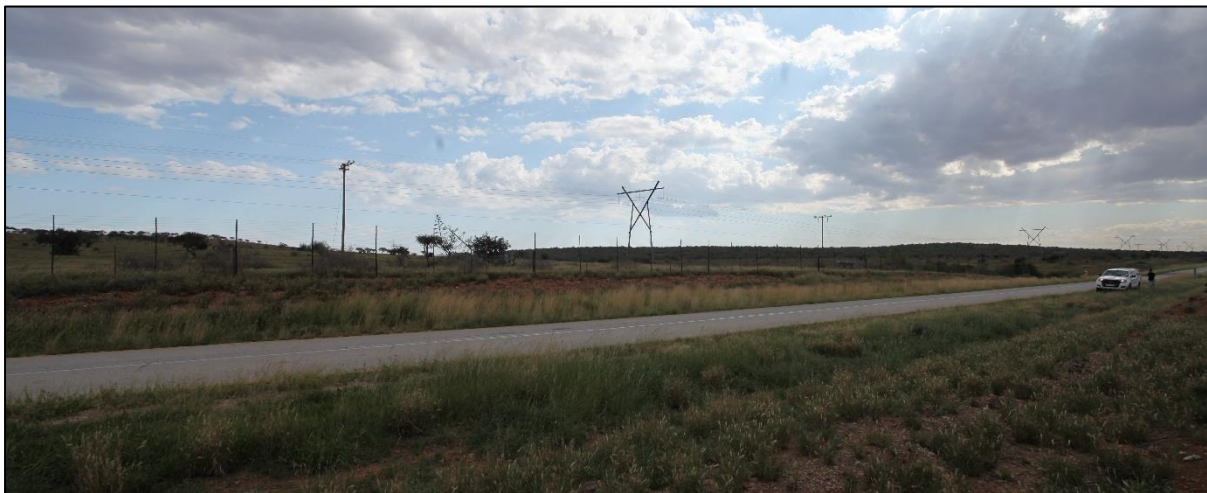
Figure 12: View from the R75 road located directly adjacent to the proposed OHPL. As is evident on the photograph, the existing overhead powerlines fades in the distance the further the structures are from the observer. The proposed OHPL will therefore not be significantly visually intrusive to motorists traveling along the R75, and it will not be noted as the visual impact is already present.
