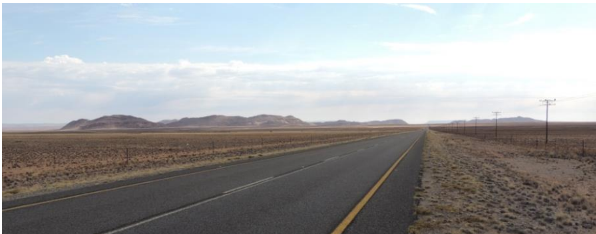
Figure 19: Photograph of the N14 National Road northbound just before Aggeneys town.
