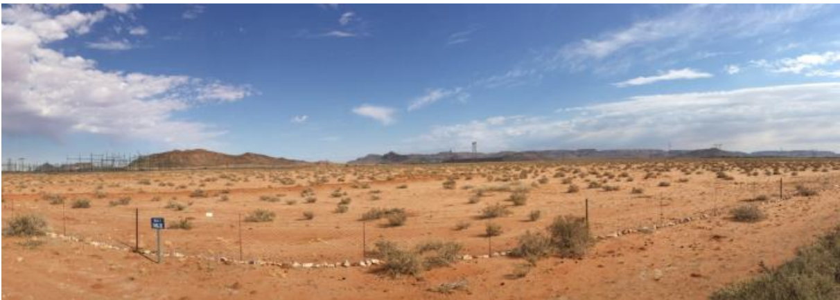
Figure 23: Photograph of the Eskom substation and town of Aggeneys as seen from the N14 National Road south of Aggeneys.
