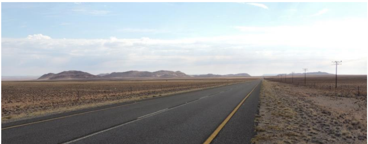
Figure 15: Photograph of the N14 National Road northbound just before Aggeneys town.
