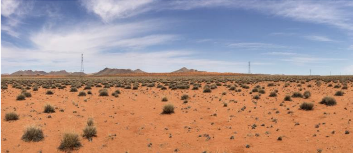
Figure 18: Photograph of the Eskom 220kV power line as seen from the proposed southern CSP site.
