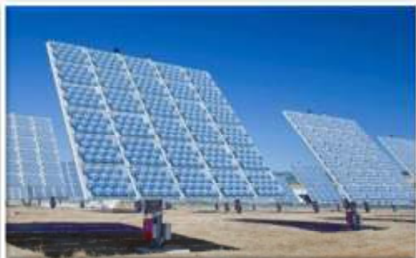
Example of CPV-type solar panels (Source: www.ecofriend.com )
