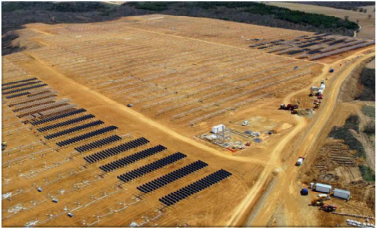
Figure 13: De Aar Solar Capital Energy Project ( www.solarcapital.co.za )
