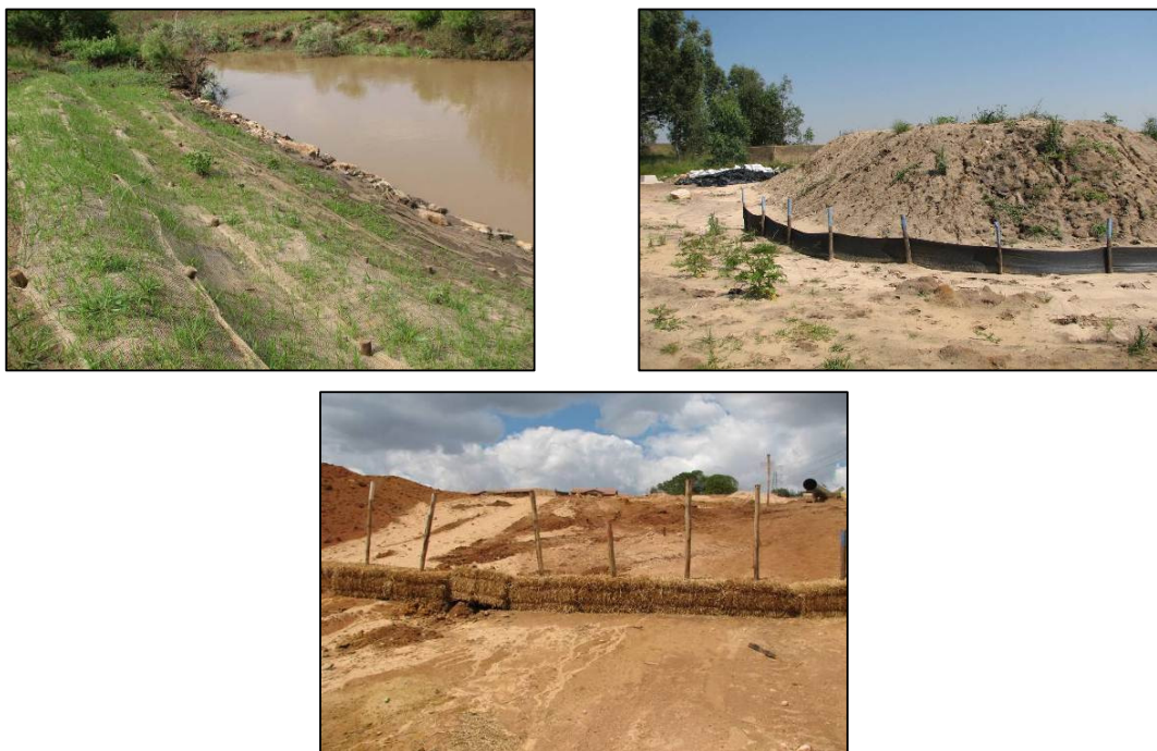
Figure 32: Typical soil erosion mitigatory measure: BioJute Installation ( top left ); a silt fence protecting a stockpile ( top right ) and pegged hay bale wall used to reduce runoff velocities ( bottom )
