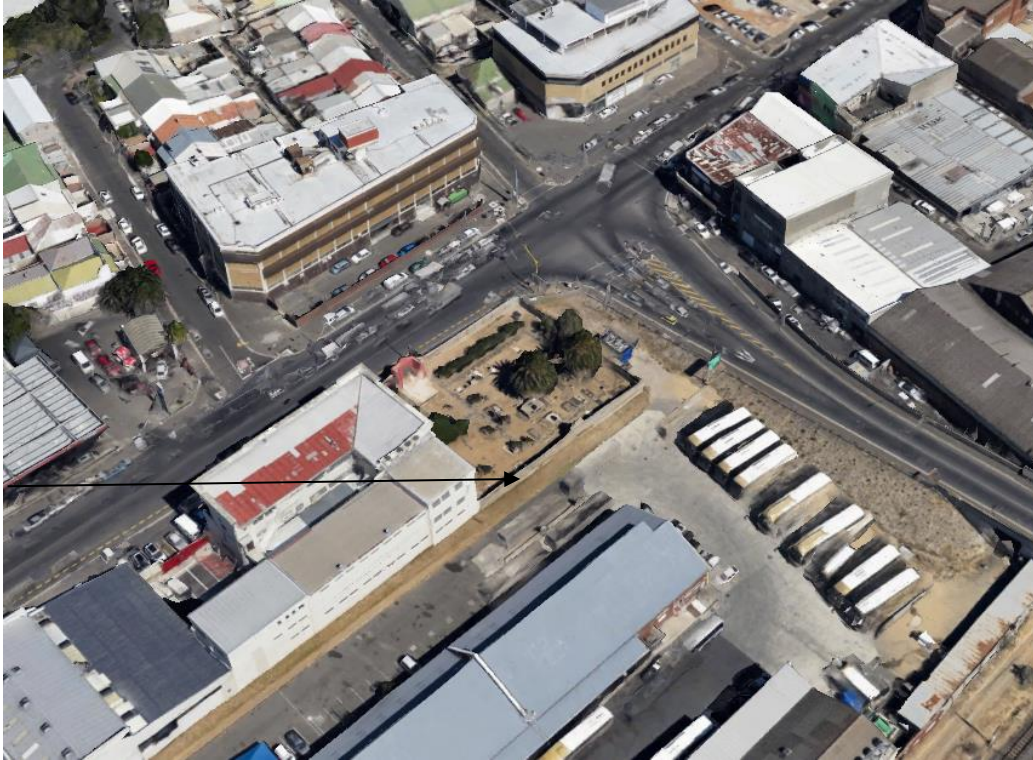
Fig 4. The northern boundary wall which requires repair rebuilding and a security fence.
