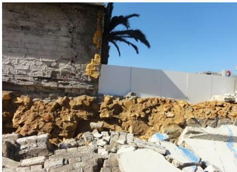
Fig 15 temporary boarding in place July 2018.
