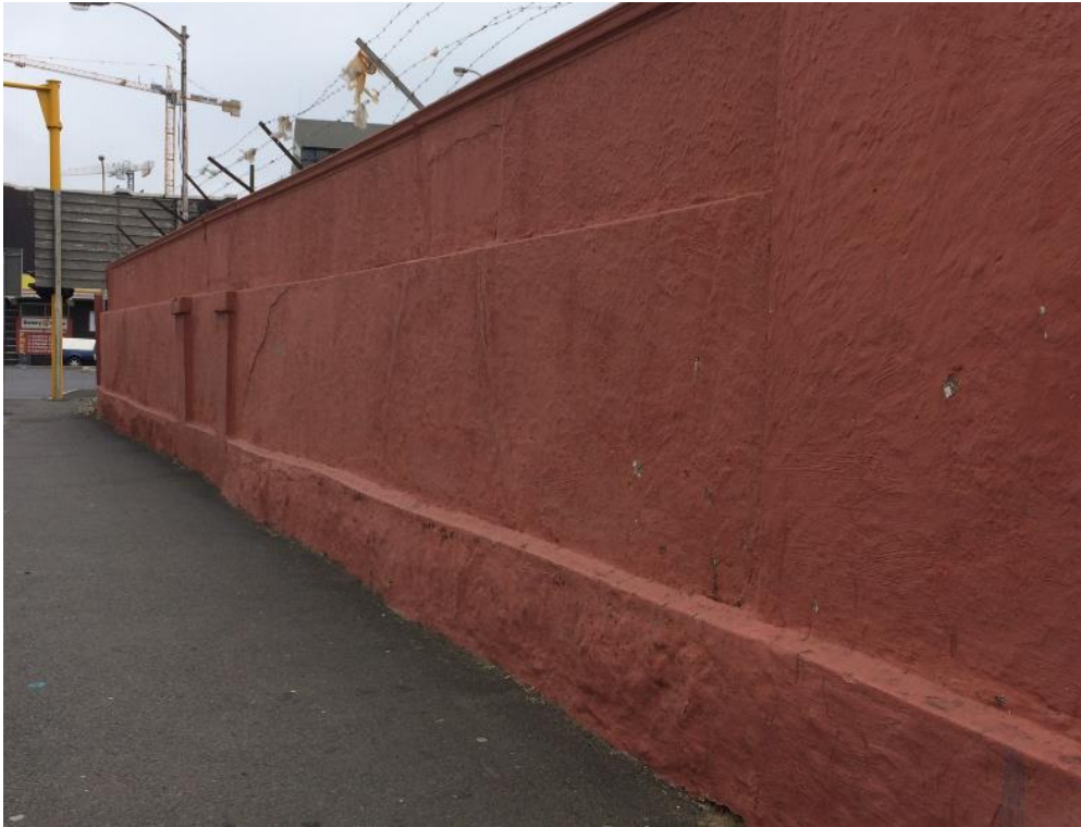
Fig 7. The cemetery walls with a stone base plastered early walls and raised height. Also shown is a potential earlier entrance.
